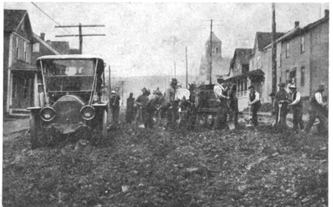
Road Makers Preparing the Way at Johnstown.
